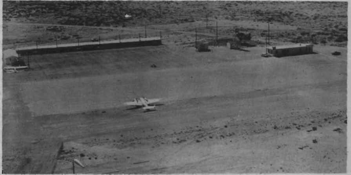
DESERT AIR FIELD - Dwarfed by the expanse of desert, the operations building, right, at Condron Field looks much less than its 100 feet long and 20 feet wide. Barely visible behind the building is a 75-foot forest ranger tower modified for traffic control. Structures at left are shop and hangars belonging to the White Sands Missile Range Flying Club. Plans are underway for paving a runway at the historic air field that lies in a dry lake bed and atop an Indian burial ground. (U.S. Army Photo)
